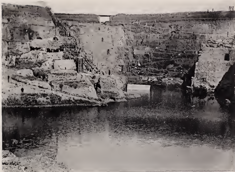
FIG. 1.—N. E. CORNER OF KODUR MANGANESE-QUARRY.
